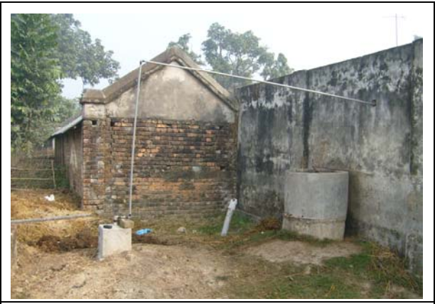
Overhead Gas distribution line
