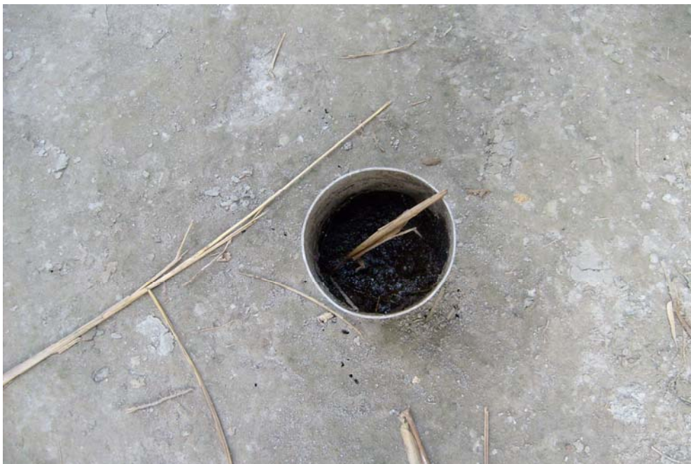
Picture 3: An extra pipeline for connecting with toilet to add night soil in future
