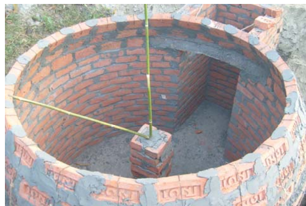
An under constructed plant
