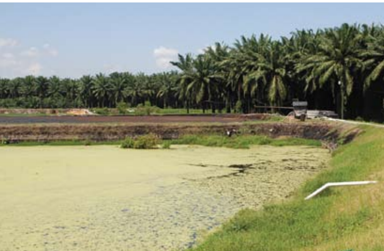
Waste water treatment at HONDUPALMA. El Negrito, Yoro.
