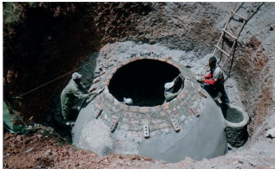
Figure 13. Fixed-dome biogas digester under construction in Kokebe Tsebah School
