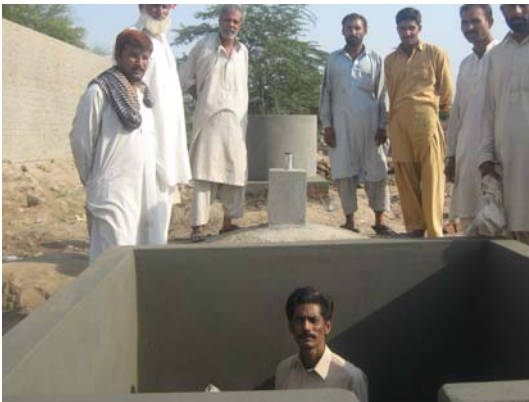
Photograph 4-15: Construction of Slurry pit in progress
