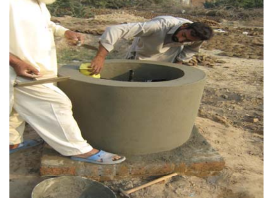
Photograph 4-12: Compartment for feeding of animal manure being completed
