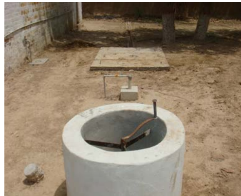
Photograph 4-16: Feeding compartment, biodigester unit outlet and slurry pit (with lid) on completion of biogas unit
