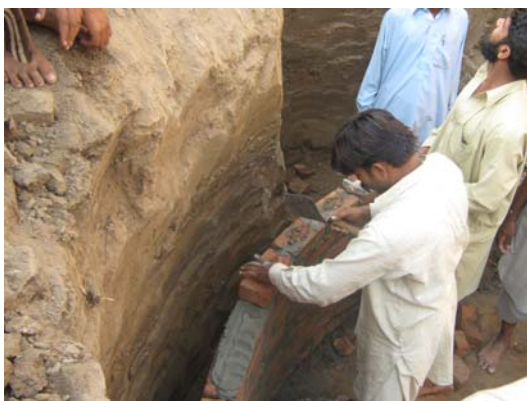
Photograph 4-5: Wall of biogas unit being constructed from bricks
