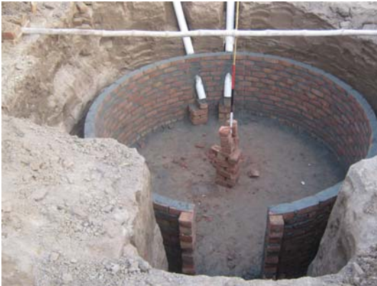
Photograph 4-7: Brick wall of the biodigester unit completed
