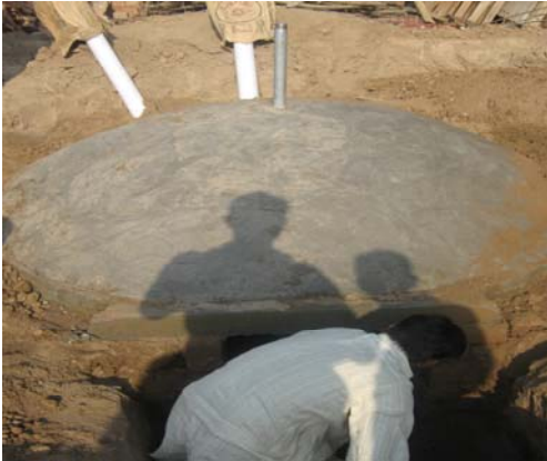
Photograph 4-13: Biodigester unit completed with concrete dome
