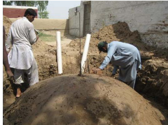
Photograph 4-8: Dome of the biodigester unit constructed
