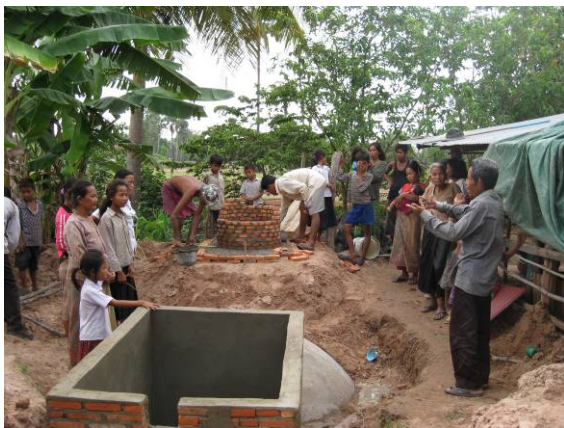
A under-construction biodigester
